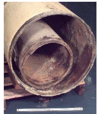
Full Bore Pipeline Failure
